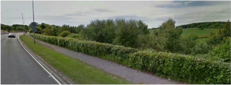
FIG 3 Existing woodland and hedging along A92 Road.
